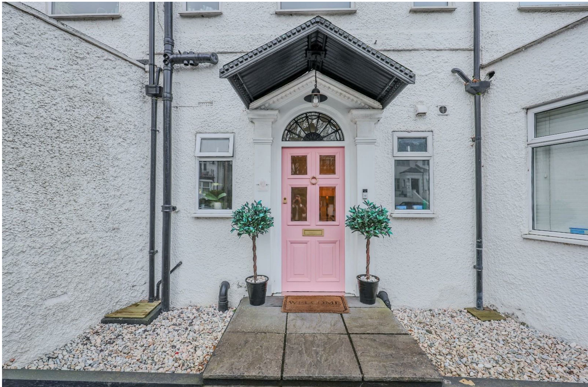
Kings Road, Westcliff-on-Sea £425,000
